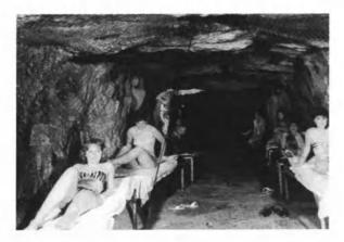
Fig. 8.74. Treatment station No. IV in the Böckstein heat gallery. Distance of entrance 2 238 m, air temperature 41.5 °C, humidity 99%
